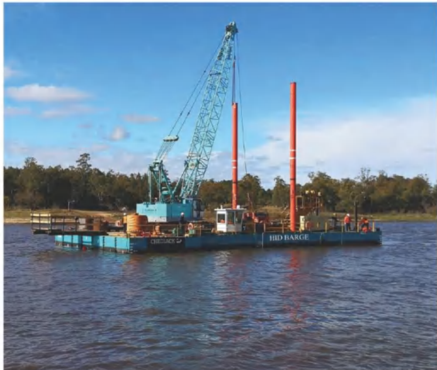
Uruguay 2019 Crane Barge Bridge Building
